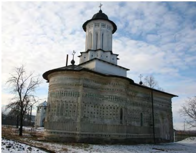
Figure 2. Aroneanu Church – exterior view
