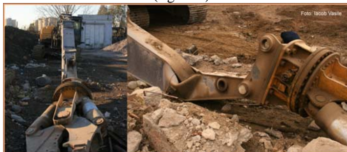
Figure 5. Hydraulic scissors arm of 21 m damaged
