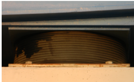
Figure 11. LRB bearing from Basarab passage
