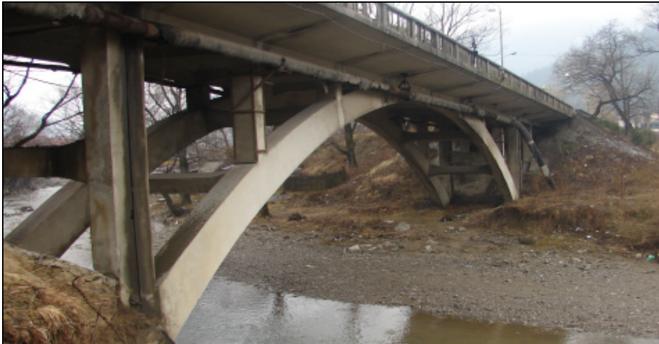
Figure 1. View of bridge on national road at Bicaz
