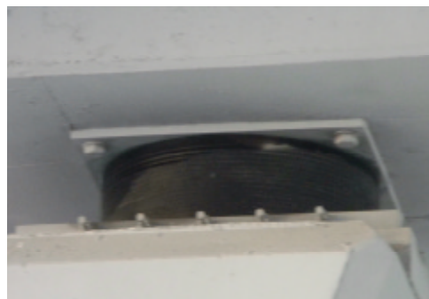
Figure 9. HDRB bearing from Basarab passage
