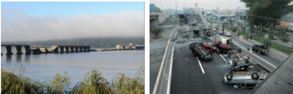
Figure 2. Puente Viejo Pedestrian Bridge (the Veijo Bridge was restricted to pedestrian traffic two years before the earthquake) [4]; Figure 2. Bridges destroyed by the earthquake dated February 27, 2010 from Chile (8.8 degrees on the Richter scale, it lasted 9s, took place at a depth of 13km and was followed by 2 aftershocks bigger than 5 degrees) [5]
