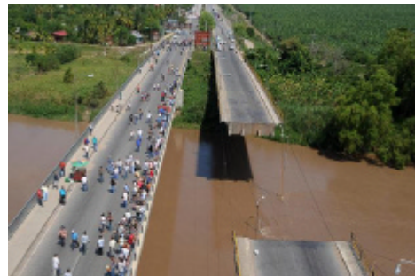
Figure 5. Seongsu bridge from Seoul (South Korea) having a total length of 1160m, crashed on October 21, 1994 [7]; Figure 6. “La Democracia” bridge erected in 1963 over Uluá river, crushed during an earthquake of 7.1 degrees on the Richter scale [8]
