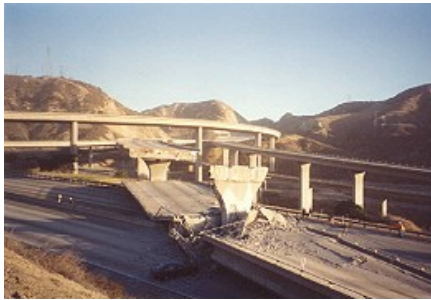
Figure 3. Crash of bridge decks at the motorway intersection way, earthquake Northridge Earthquake, January 17, 1994, California, 6.8 degrees on the Richter scale [6]; Figure 4. Crash of a bridge pile because of the insufficient confinement reinforcements, earthquake Northridge Earthquake, January 17, 1994, California, 6.8 degrees on the Richter scale [6]
