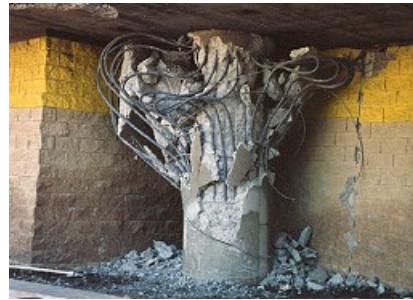
Figure 3. Crash of bridge decks at the motorway intersection way, earthquake Northridge Earthquake, January 17, 1994, California, 6.8 degrees on the Richter scale [6]; Figure 4. Crash of a bridge pile because of the insufficient confinement reinforcements, earthquake Northridge Earthquake, January 17, 1994, California, 6.8 degrees on the Richter scale [6]
