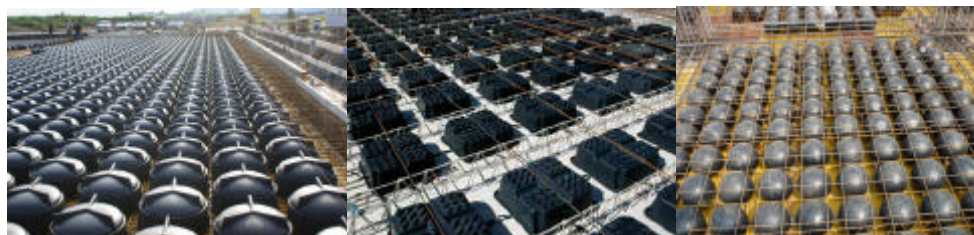
Fig. 1 Details of constructive systems for reinforced concrete floor with bell-shaped, cubic and spherical voids
