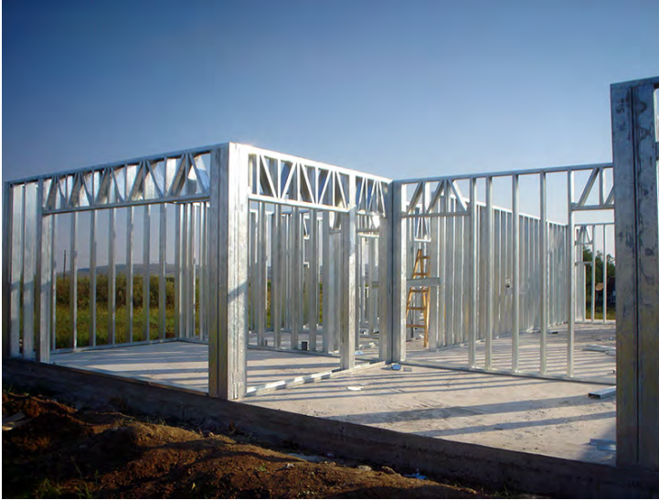
Figure 1. Structure made of light-gauge steel profiles
