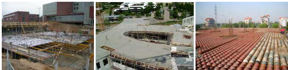
Figure 16. Aspects during casting in place of the concrete slab with spherical gaps
