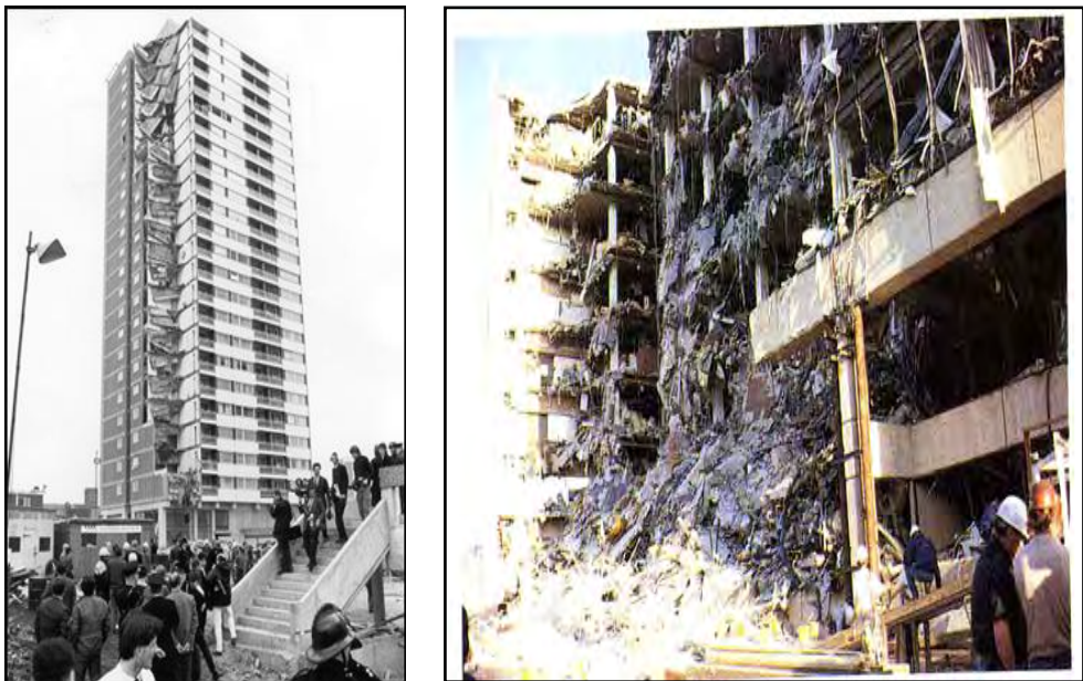
Figure 1. Failure boundaries in the Roman Point apartment building [2] and in the A.P Murrah Federal Building [3]
