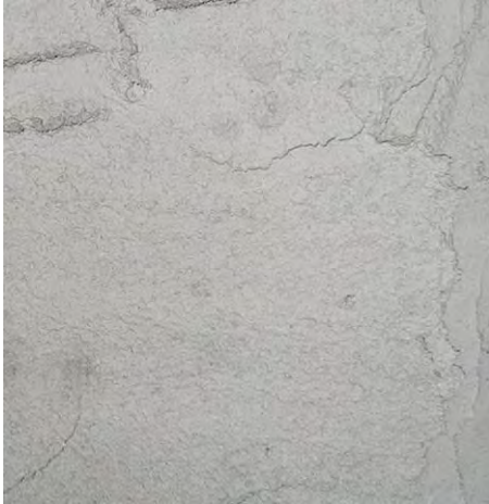
a) Specimen of plaster of referential
