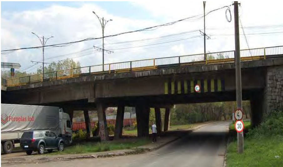
Figure 1. Lateral view towards the first hit beam
