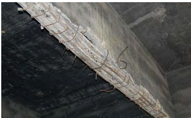
Figure 4. Beam 2 (central beam)
