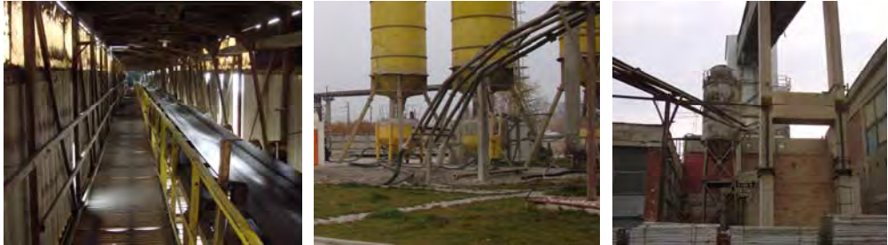
Fig.2.5. (a) conveyor belt, (b) cement pipes for transport, (c) station for concrete preparation
