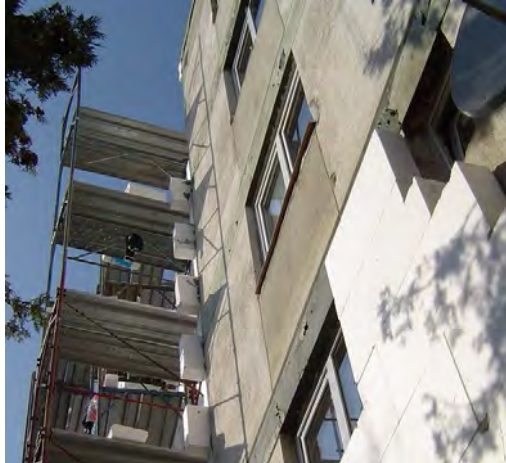
Figure 5. Building from Cluj- Napoca town in the process of rehabilitation with 15 cm of polystyrene EPS
