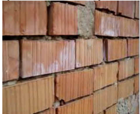
Figure 6. Efflorescence in the brickwork
