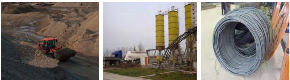
Fig.2.2. (a) storage of aggregates, (b) cement storage silos,(c) storage of concrete steel
