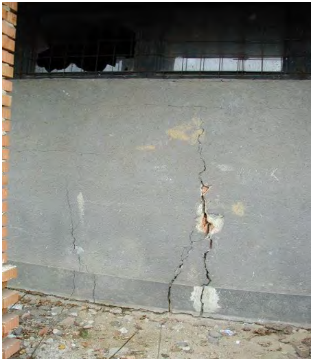
Figure 1. Cracking in the brickwork
