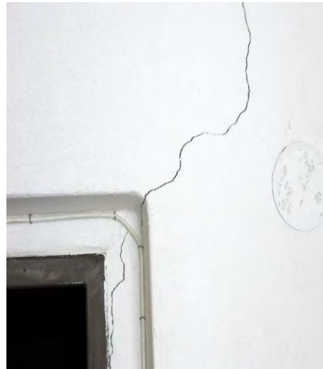
Figure 2. Cracking in the brickwork
