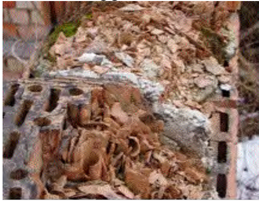
Figure 5. Brickwork of perforated bricks showing frost damage
