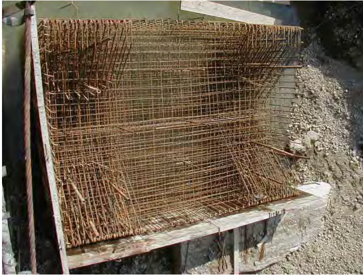
Photo 1. Widening of a bridge to fulfill the actual traffic requests
