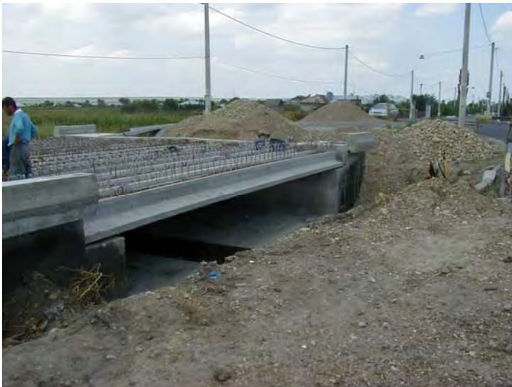
Foto 2. Replacement of an existing small bridge
