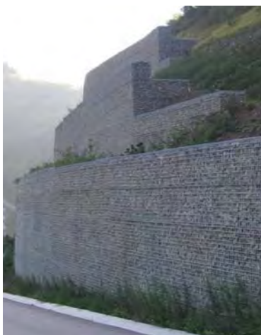
Figure 2. Retaining wall of Textomur with vertical mineral facing
