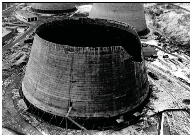
Fig. 1 RC Cooling tower after the collapse
