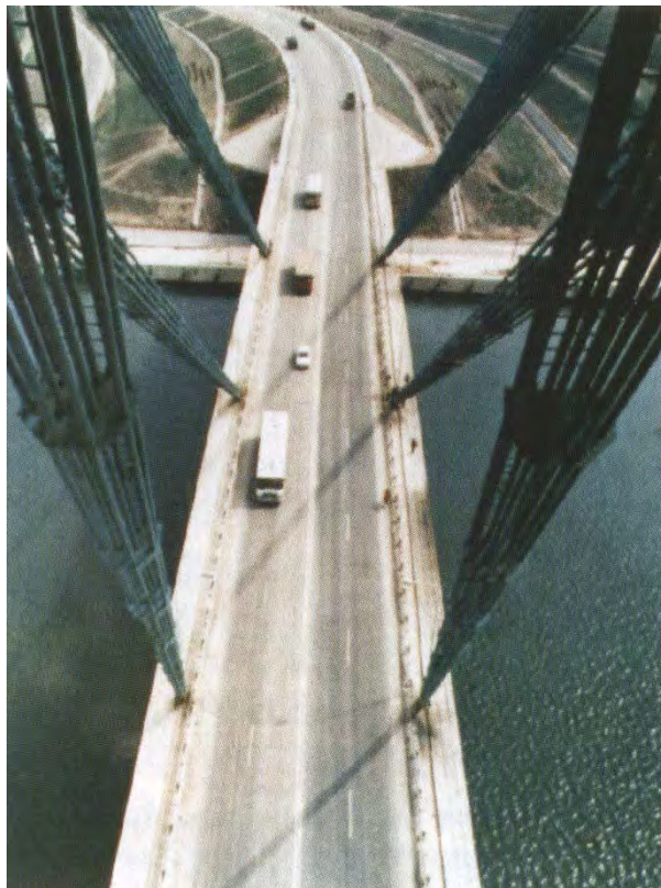
Figure 1. The Agigea Bridge from Romania
