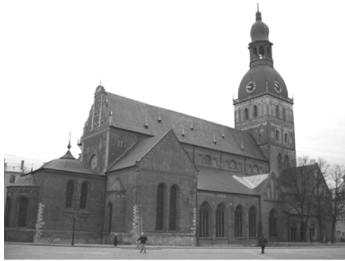
Figure 1. North front of Riga Cathedral
