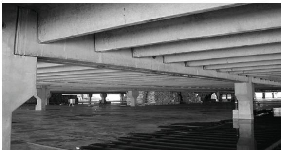
Fig. 2 – Shown Precast concrete beams with installations holes.
