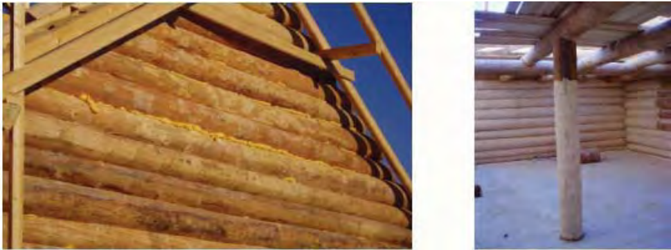
Figure 1. Left –Incorrect construction and insulation of gable; Right –Incorrect placing of vertical element (an adjusting screw is missing)
