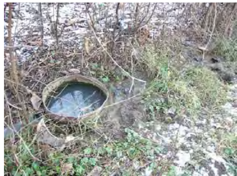
Photo 4. Malfunctioning of the drainage pipeworks due to the mass movement
