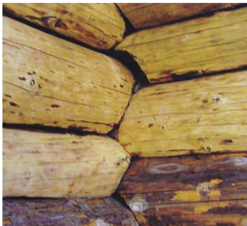
Figure 2. Incorrect corner structure (roughly encircled shapes)
