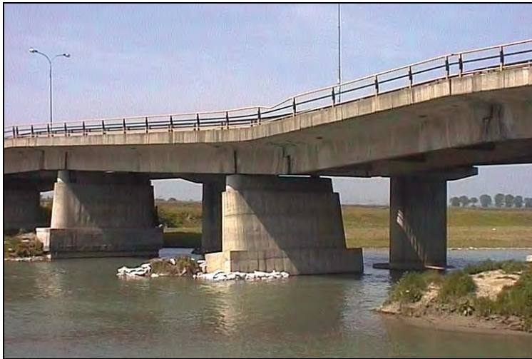
Fig.1. Technical state of one of the bridges over Moldova river after infrastructure’s erosion
