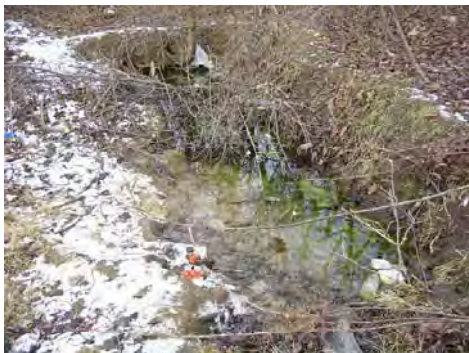
Photo 3. The water bogging along the slope due to the soil mass movement
