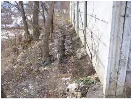
Photo 1. Landsliding phenomena at the upper side of the sport field
