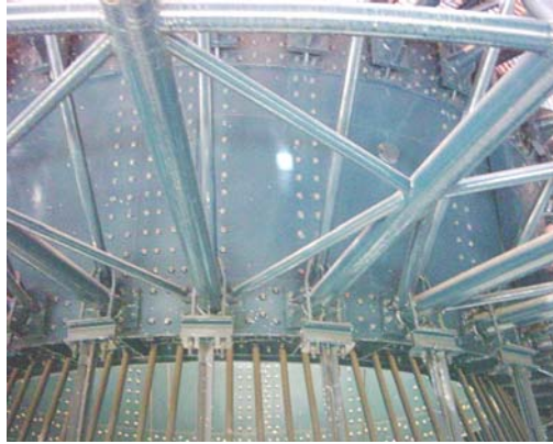
Figure 4 – View with the connection between the bottom flanges of the semi-arches at the central ring
