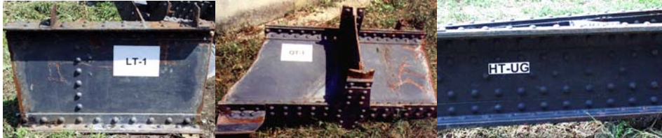
Figure 7 Stringer, cross girder and main girder pieces
